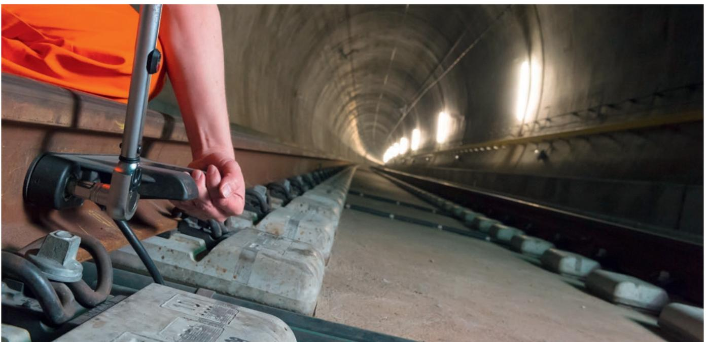
Installing a Sk30K wheel sensor in the Swiss Gotthard base railway tunnel; the longest railway tunnel in the world
