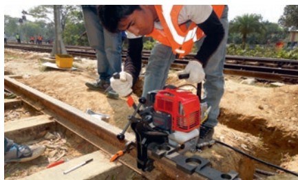
Drilling of the hole
